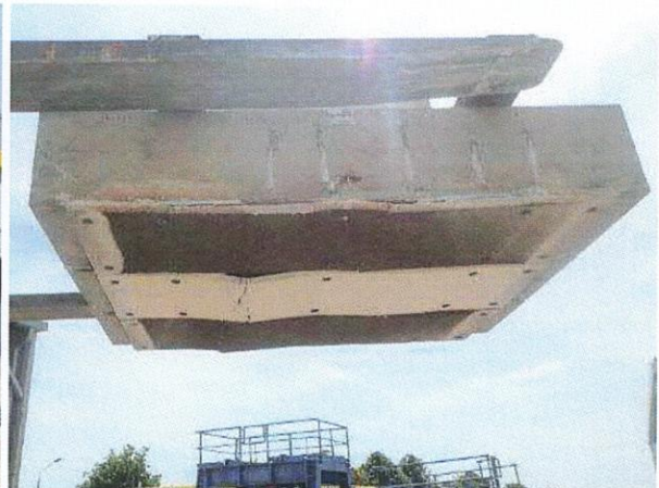
Photo A3-15 View of cracked fire protection panels directly after the fire test
