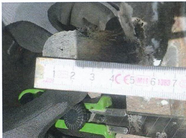
Photo A3-18 Section of joint material from joint 2
