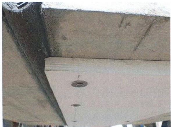
Photo A3-4 Fastening of the Promatect-T fire protection panel
